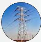
Electrical Power Supply
