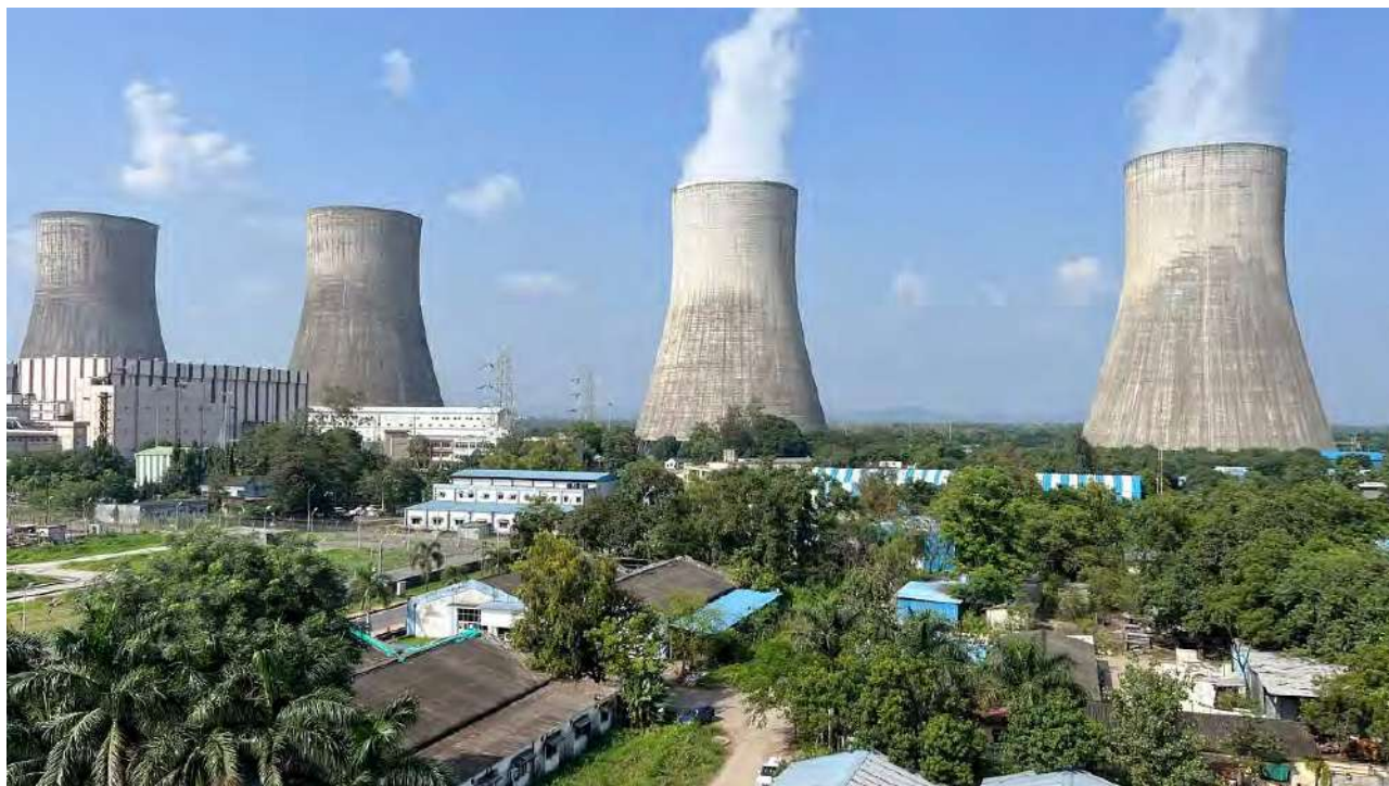
A view of India's first indigenously developed 700-megawatt electric nuclear power reactor that has been established at the Kakrapar Atomic Power Station.
